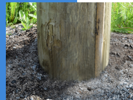
BACKFILL & TAMP
